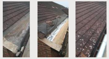
RIS Contract Services carried out the Roofing, Fire Protection and Scaffolding Works at the Swan Court Nursing Home in Milton Keynes on behalf of one of our Clients. Once the Scaffolding was erected Safely, the works consisted of removing 3x Roof tiles to carry out Fire Protection works the reinstating the Roof tiles with no disruption. The job was a real success and earnt us another 6 Nursing Homes around the Southeast and Midlands.
